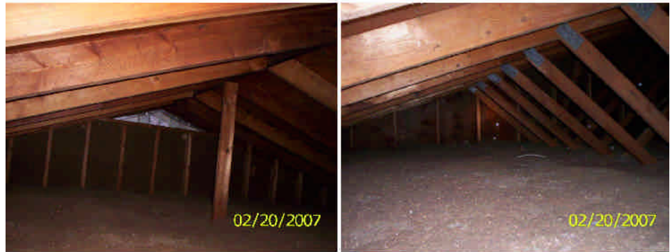
East attic view (L) -- West attic (R)
