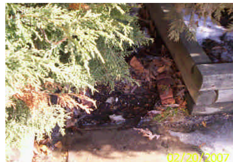
Driveway drain on east side of drive.
