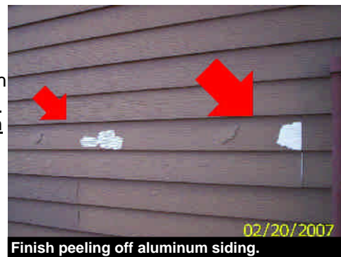
Finish peeling off aluminum siding.
